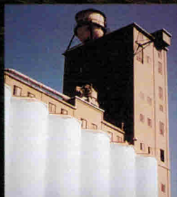
Manufacturing Plant, Iowa
